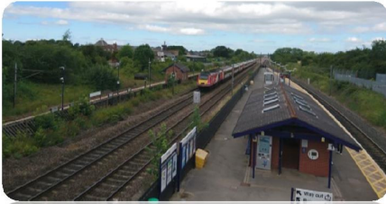
Below: Thirsk Train Station
